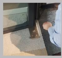
By modifying the power setting, and adjusting the closing speed, the resistance was overcome and the doors enabled to close correctly
