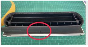
Remove the rest of the release paper and stick the intumescent around the letterplate tightly. Continue with the other intumescent as highlighted
