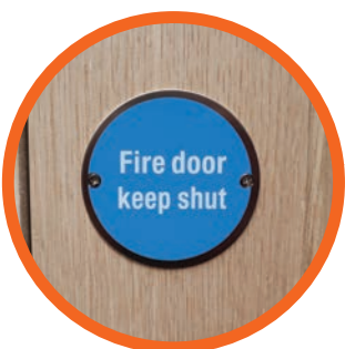
Signage e.g FDKS sign
